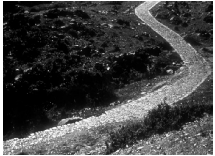
Roman Road going left and right
